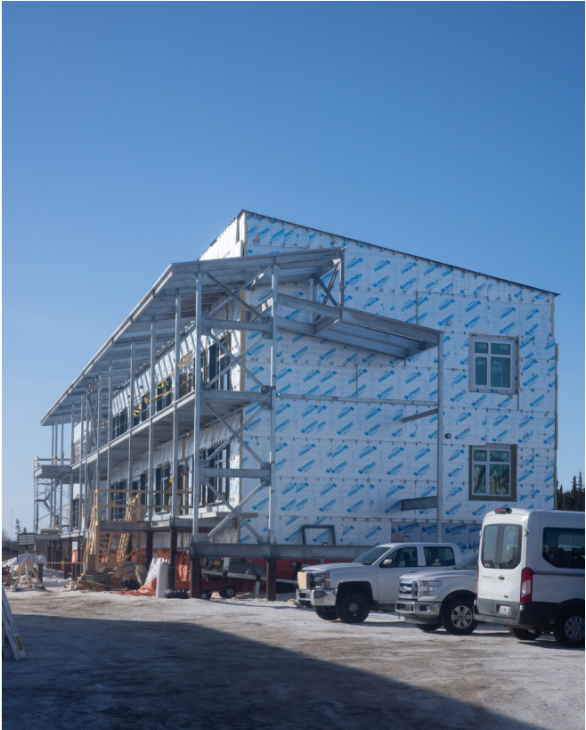
Construction continues for new Wellness Center and 10-plex.
